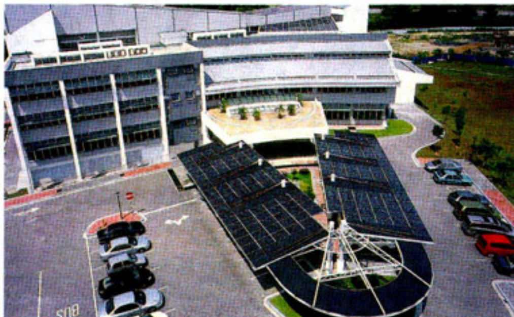
The 4,000 sq m zero energy office building not only takes advantage of free sunshine to light its interiors and produce solar power, but also relies on insulated building materials to keep out the heat.
