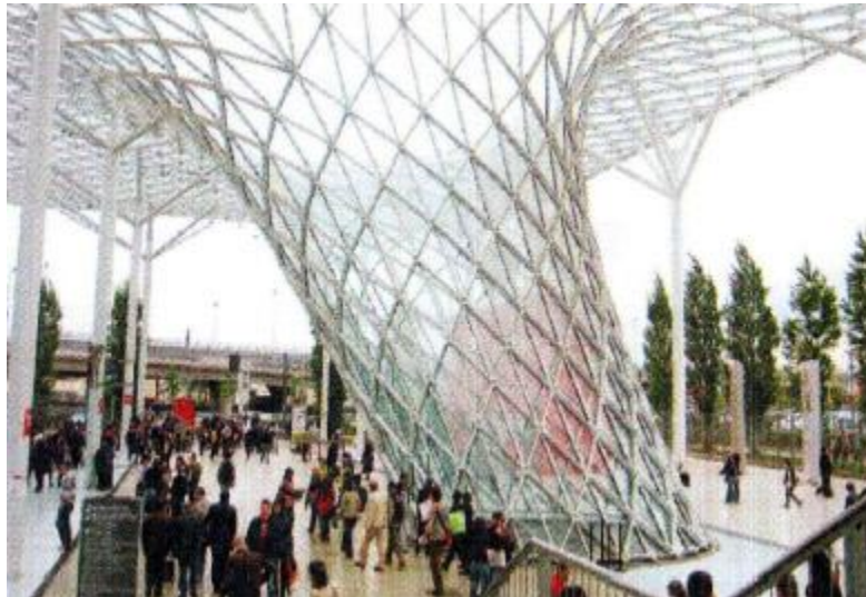
The roof at the entrance of the Milan Fairgrounds
